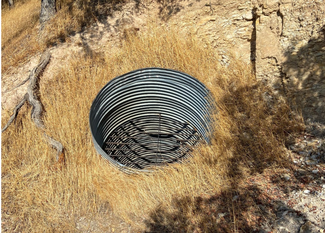
Photo 5. Close-up view of Mine entrance 3 at the Tesla Mine area.
