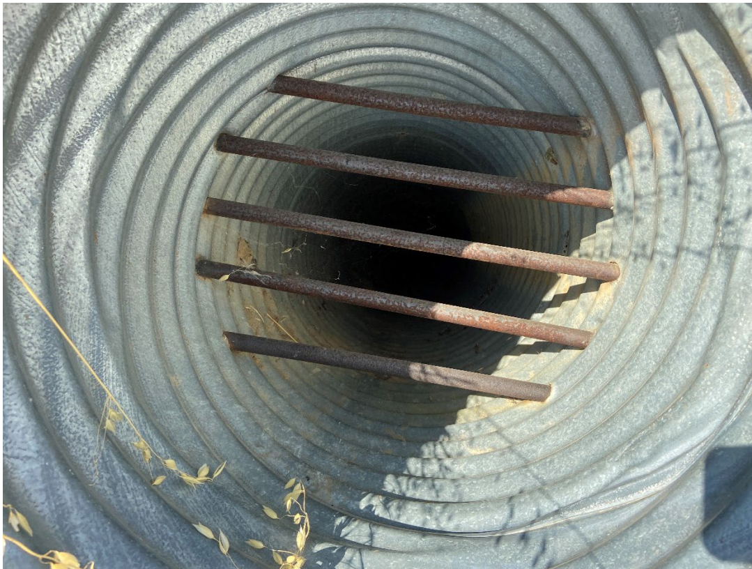
Photo 8. Close-up view of Mine entrance 5 at the Tesla Mine area.
