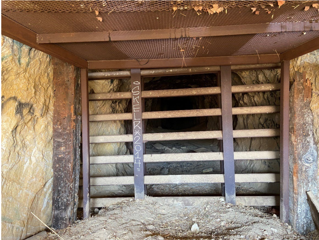
Photo 2. Close-up view mine entrance 1 at the Tesla Mine area.
